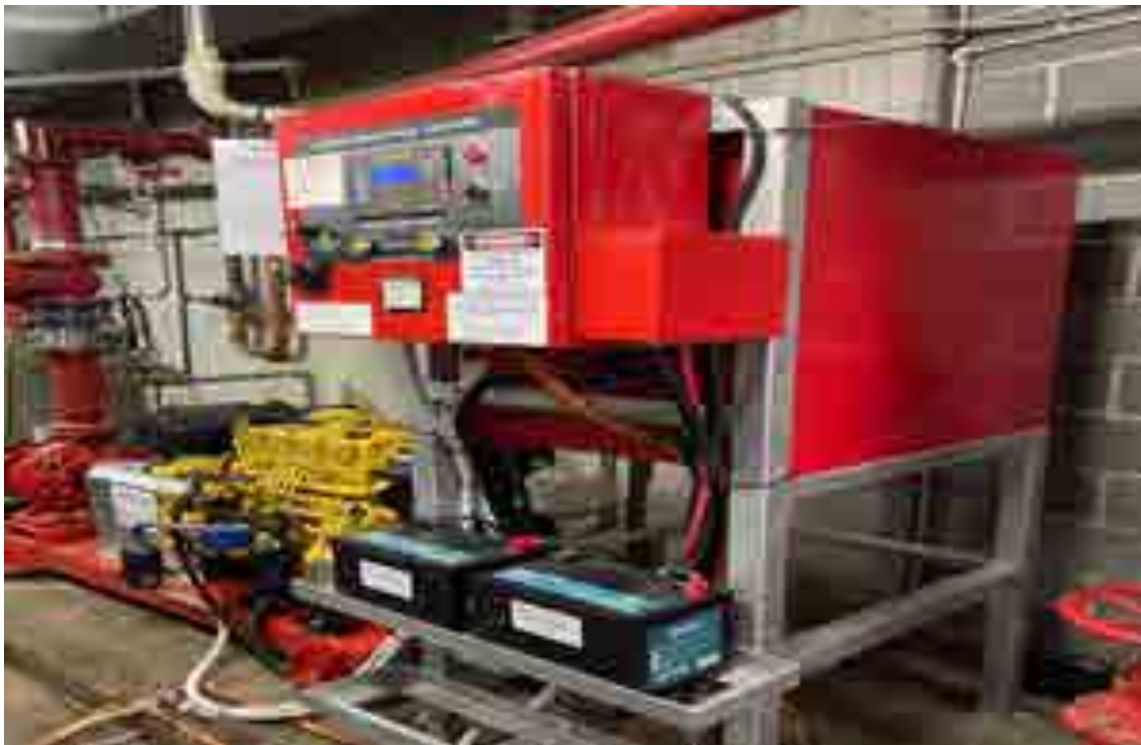
Photograph 2 Above-ground diesel tank within sprinkler / pump room
